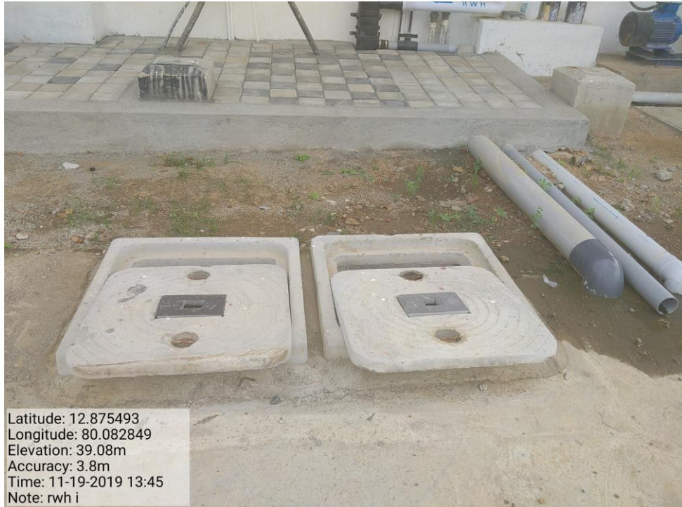
RAINWATER COLLECTION SUMP (ARCHITECTURAL BLOCK)
