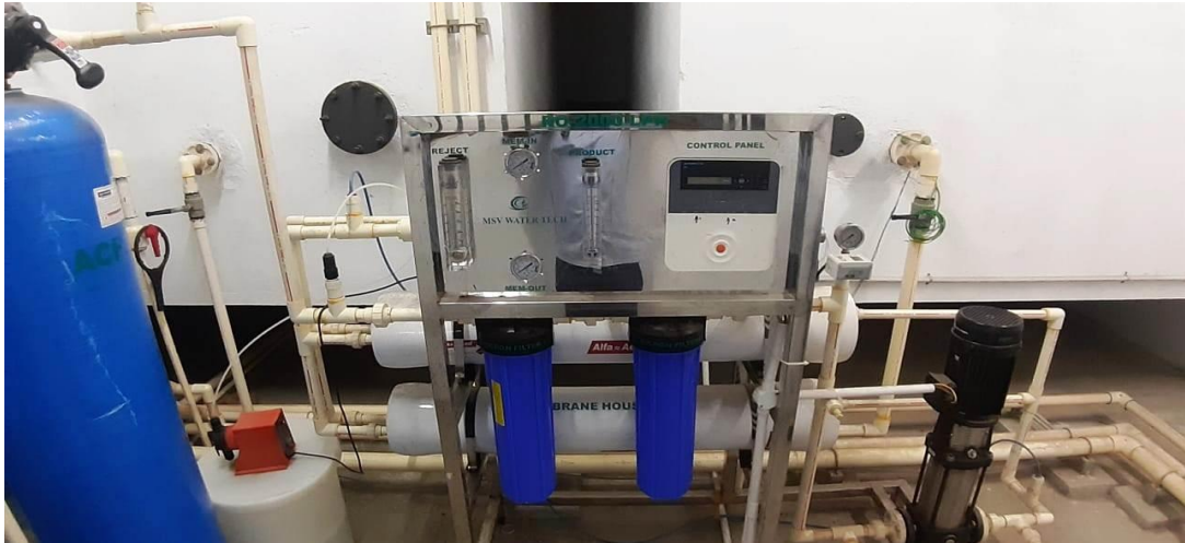
ARCHITECTURE BLOCK RO PLANT
