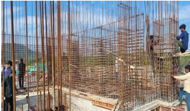
Visit to a Commercial Building at GST Road, Vandalur, Chennai on 08.05.2023
