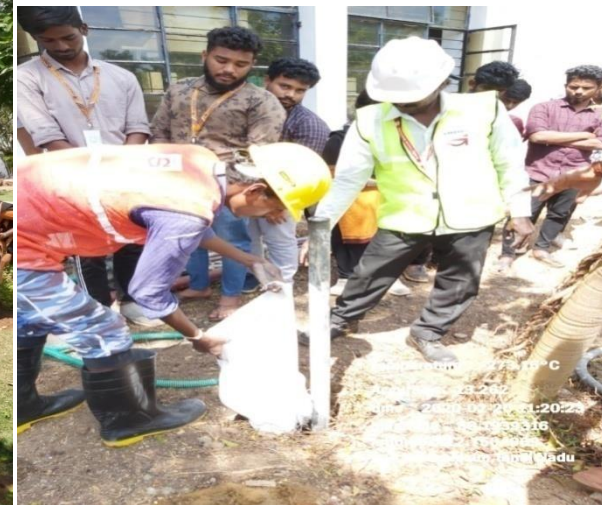
Field Visit – Lime Grouting for Soil Stabilisation – 20.02.2020
