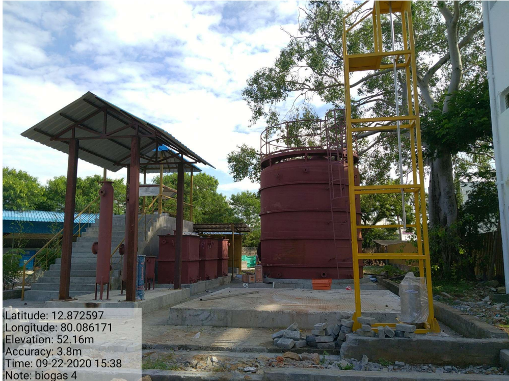
Erection & commissioning stage
