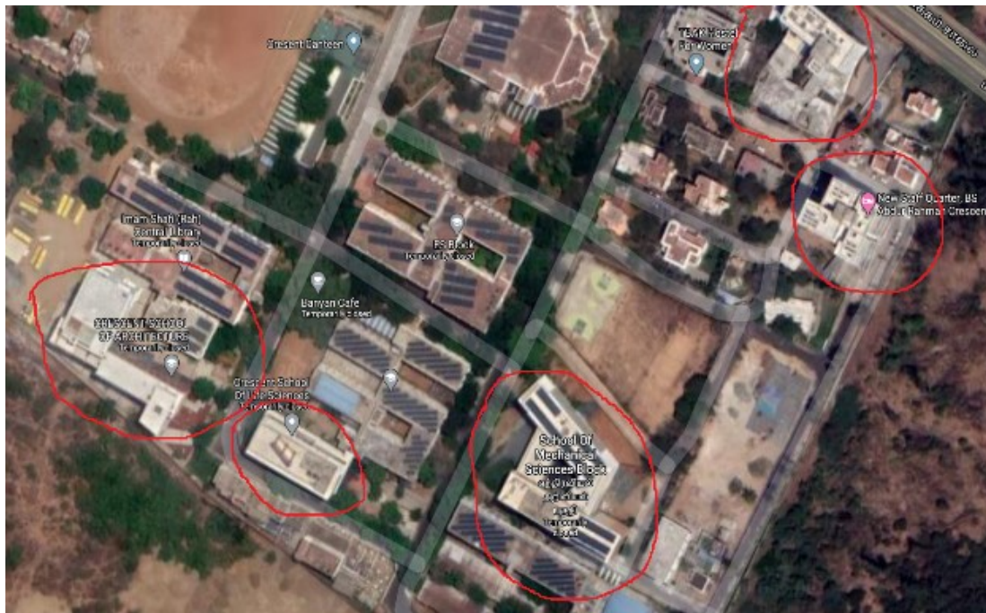
Location of Fixing up of Heat resistant roof tiles
