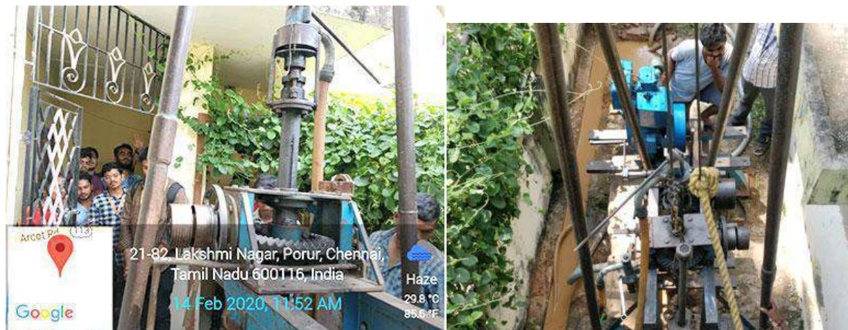
Geotechnical Investigation Camp 2020 – Porur, Chennai
