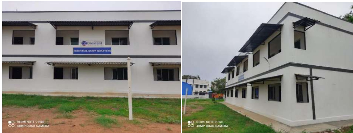
Parents Waiting Lounge and Essential Staff Quarters - GFRG Panel Affordable Housing Technique
