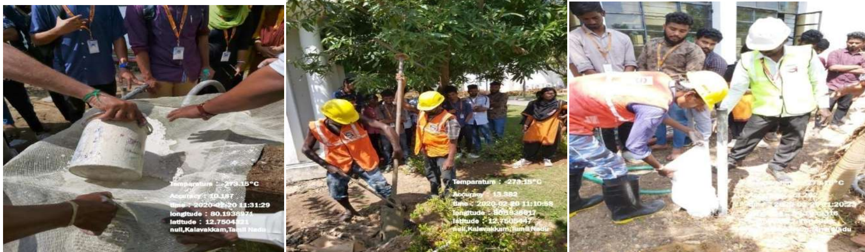
Field Visit – Lime Grouting for Soil Stabilisation – 20.02.2020
