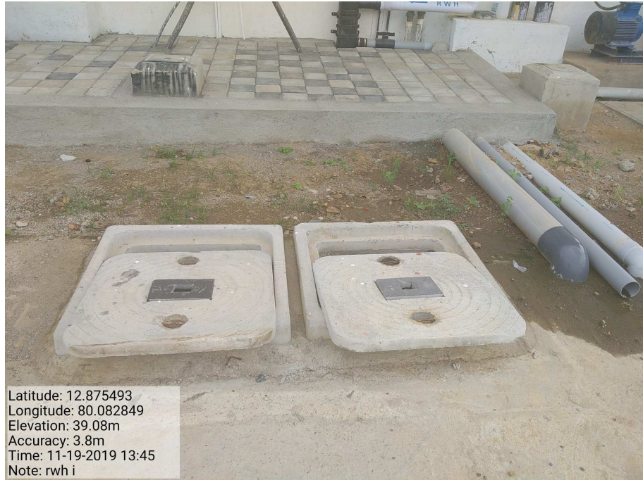
RAINWATER COLLECTION SUMP (ARCHITECTURAL BLOCK)
