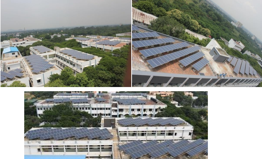
View of Roof-Top Solar Power Plants
