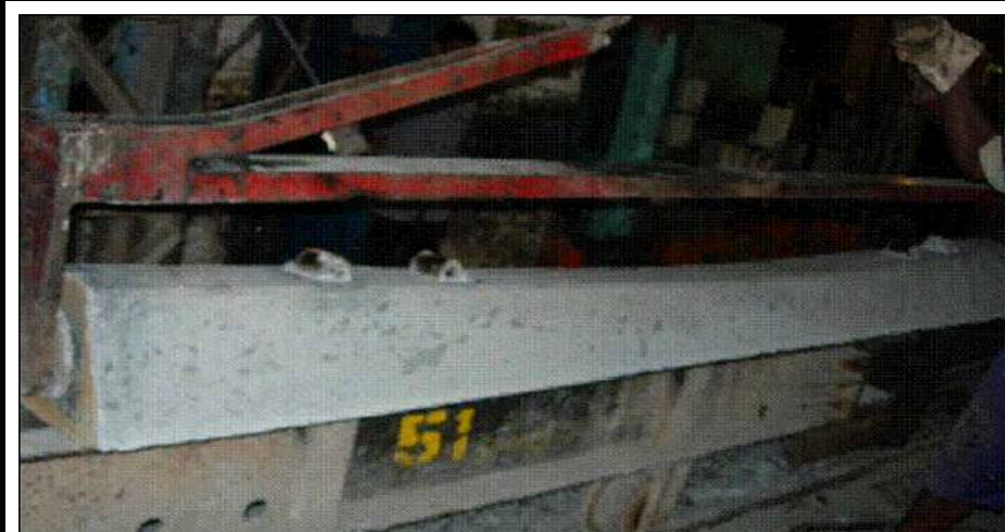
Demoulding of Sleeper
