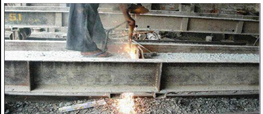
Cutting of Strands
